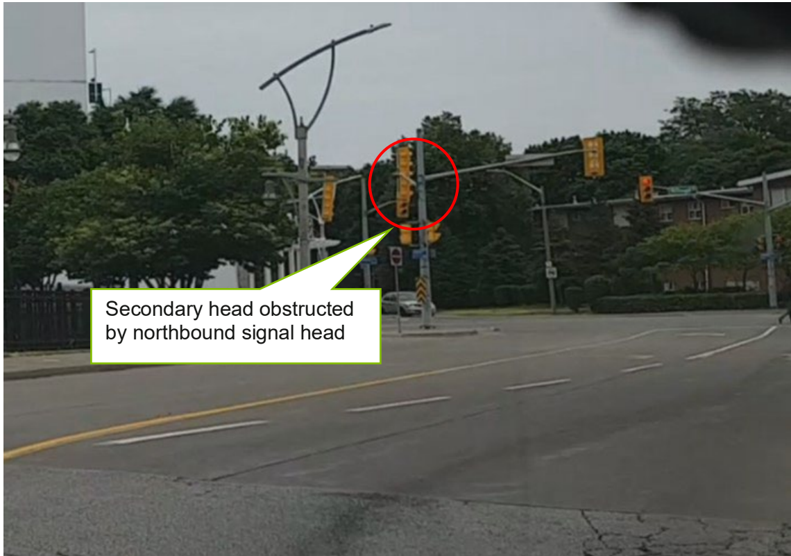
Figure 2: Eastbound Secondary Signal Head Temporarily Obstructed by Northbound Signal Head
